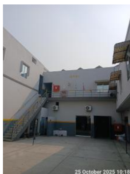
Factory building view.jpg
