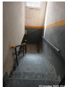
Emergency Exit Stairs.jpg
